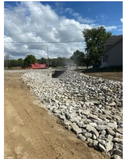
Figure 1 - Streetscape Project laying rock for drainage
